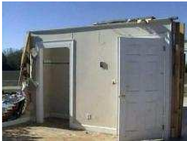
Small, interior rooms offer good protection
