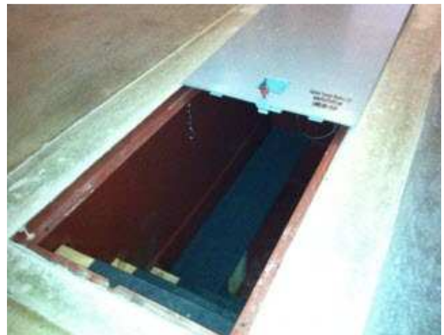
Example of a below ground tornado saferoom in a garage Courtesy Tricia Worthington
